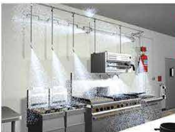
Kitchen Hood System
